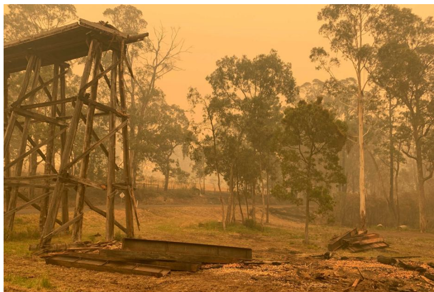
Waiwera trestle Bridge – Nowa Nowa
