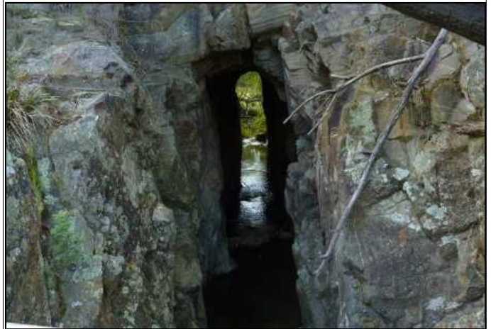
Houghtens diversion tunnel
