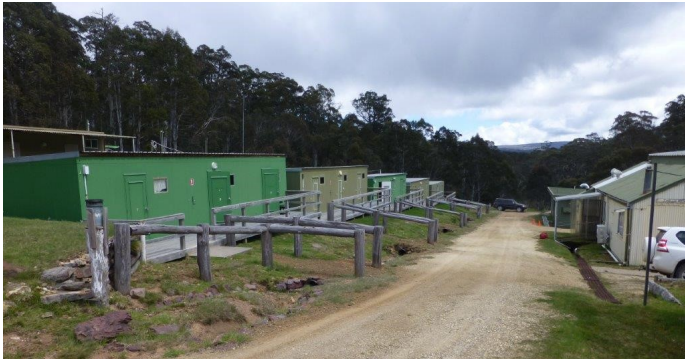
Surveyors Creek camp
